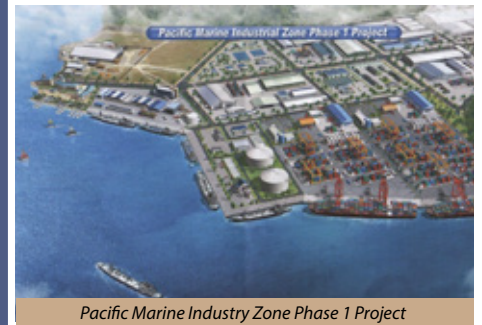
Pacific Marine Industry Zone Phase 1 Project
